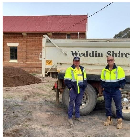
Last 2 loads of topsoil for the Memorial Garden
